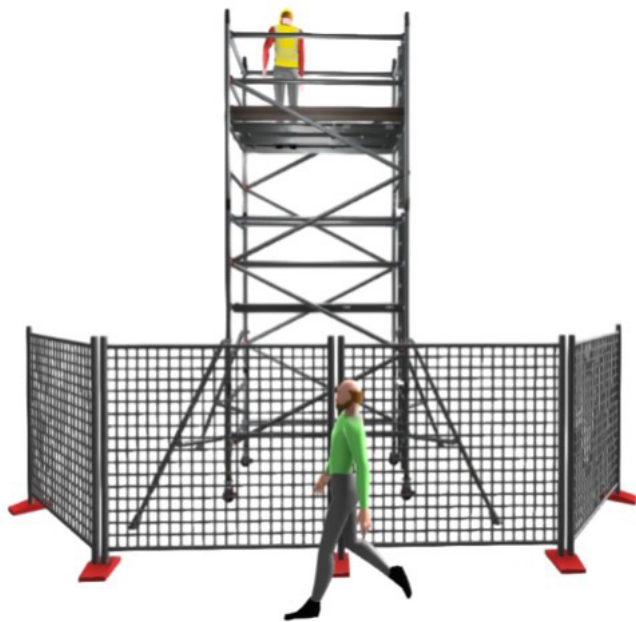
Figure 4. Erect barriers at ground level to prevent people from walking into the mobile access tower or work area. (Image credit: PASMA)
