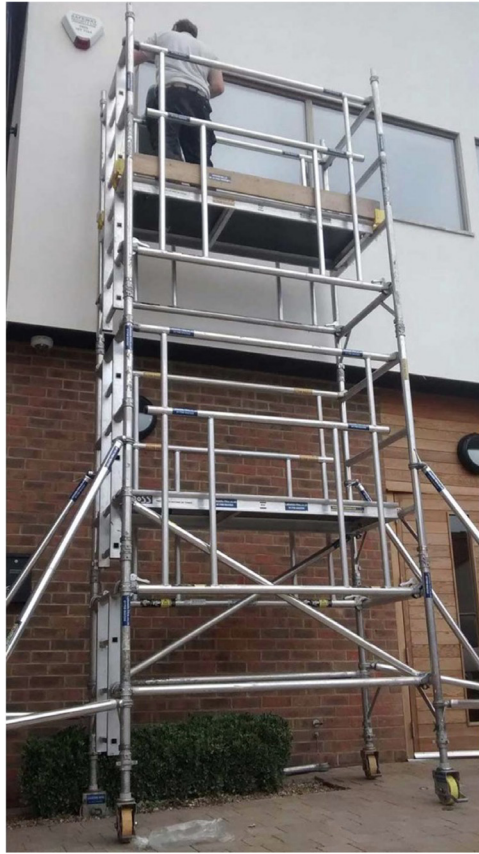
Figure 1. Mobile access towers are suitable for work at a series of locations at the same height, for example cleaning first-floor windows. (Image credit: Hire Desk)
