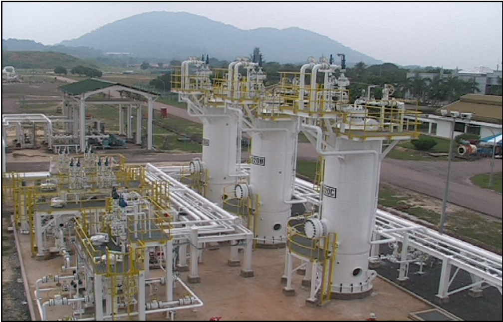
Figure 7 An example of a mercury removal system at an onshore facility
