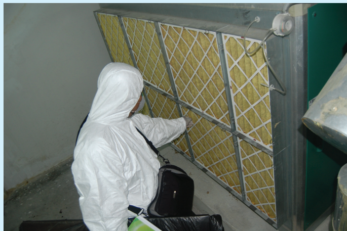
Pemeriksaan visual tahap kualiti penapis di Unit Pengendalian Udara. Visual examination for filter quality level by the Air Handling Unit.
