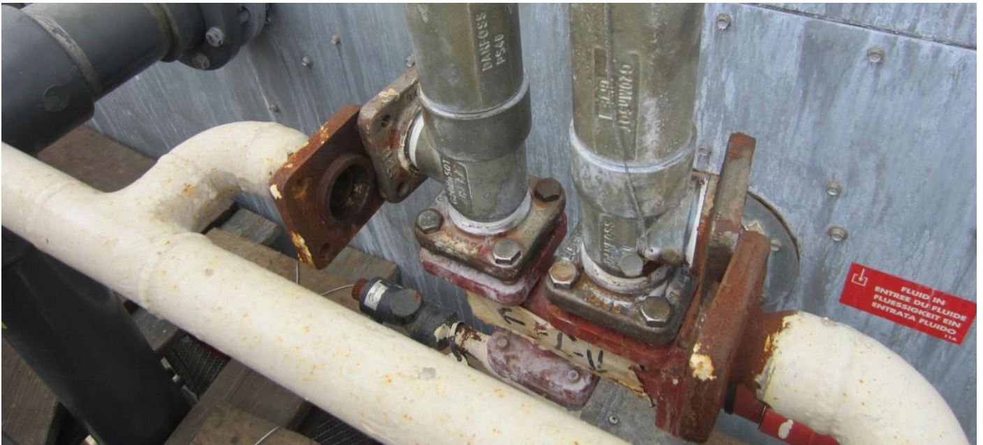
Kesan kebocoran gas toksik ammonia yang berlaku pada salah satu peralatan talian paip operasi penyimpanan gas toksik ammonia. Effects of toxic ammonia gas leakage on one of the pipeline equipment for storing toxic ammonia gas.
