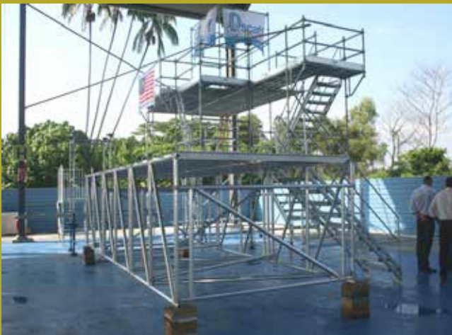
Perancah yang dipasang semasa lawatan teknikal di Dscuff Engineering Sdn Bhd Scaffolding installed during technical visit at Dscuff Engineering Sdn Bhd
