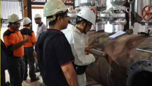
Pemeriksaan jentera menggunakan alat Positive Material Identification (PMI) Machinery inspection using Positive Material Identification ( PMI ) instrument
