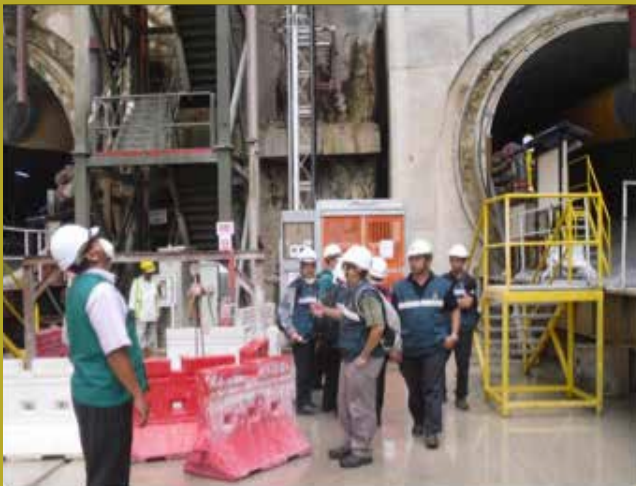
Para pegawai menjalankan penguatkuasaan KKP di tapak pembinaan terowong projek Mass Rapid Transit (MRT) Officers carrying out occupational safety and health enforcement at a tunnel construction site of the Mass Rapid Transit (MRT) Project
